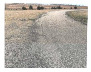
Current pavement condition is rapidly deteriorating due to water damage.
